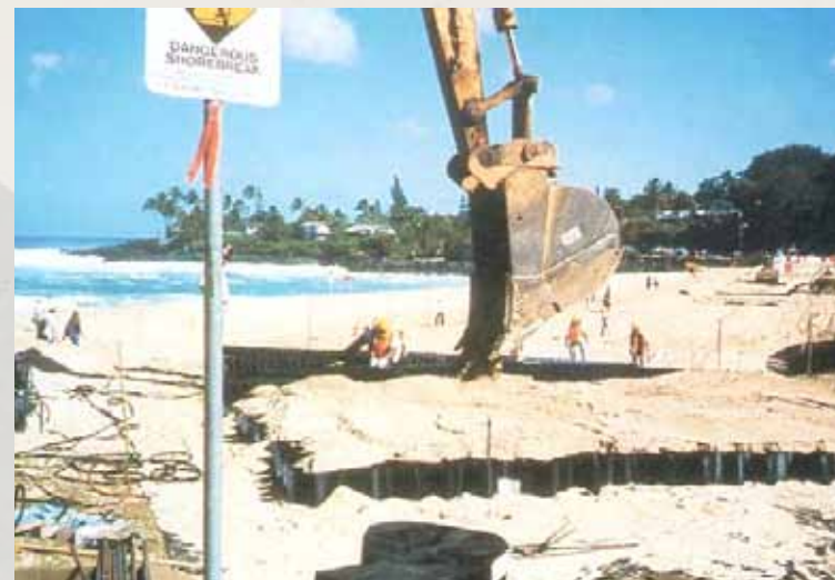
GEOCELLULAR CONFINEMENT SYSTEM BEING FILLED WITH SAND
