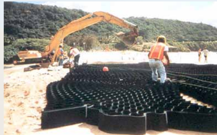
GEOCELLULAR CONFINEMENT SYSTEM BEING PLACED
