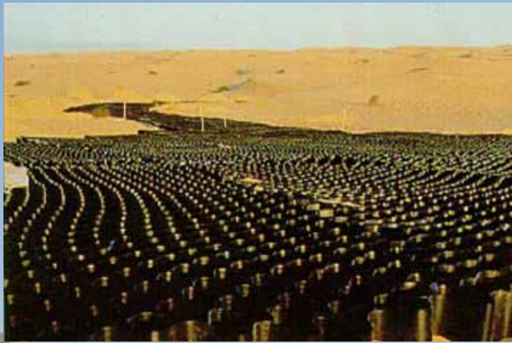
GEOCELLULAR CONFINEMENT SYSTEM AFTER PLACEMENT
