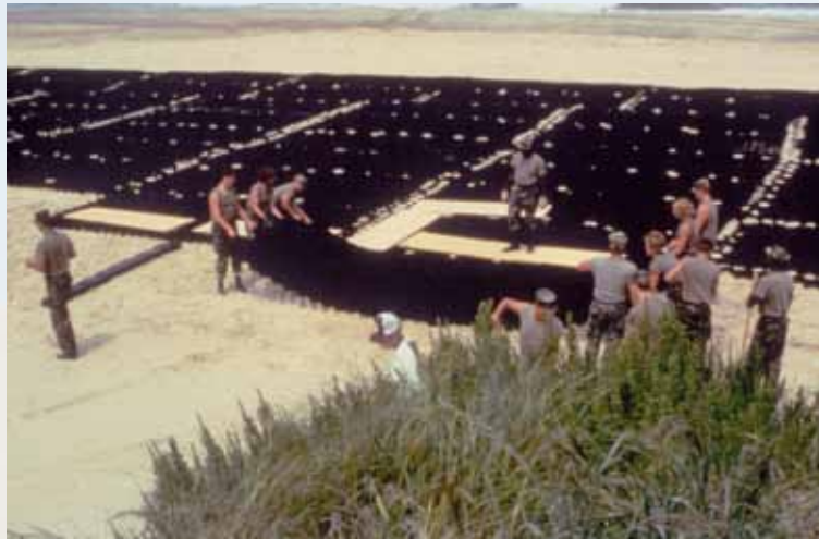
PLACEMENT OF A GEOCELLULAR CONFINEMENT SYSTEM
