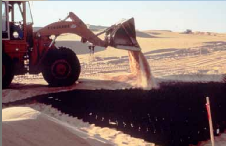
GEOCELLULAR CONFINEMENT SYSTEM BEING FILLED WITH SAND
